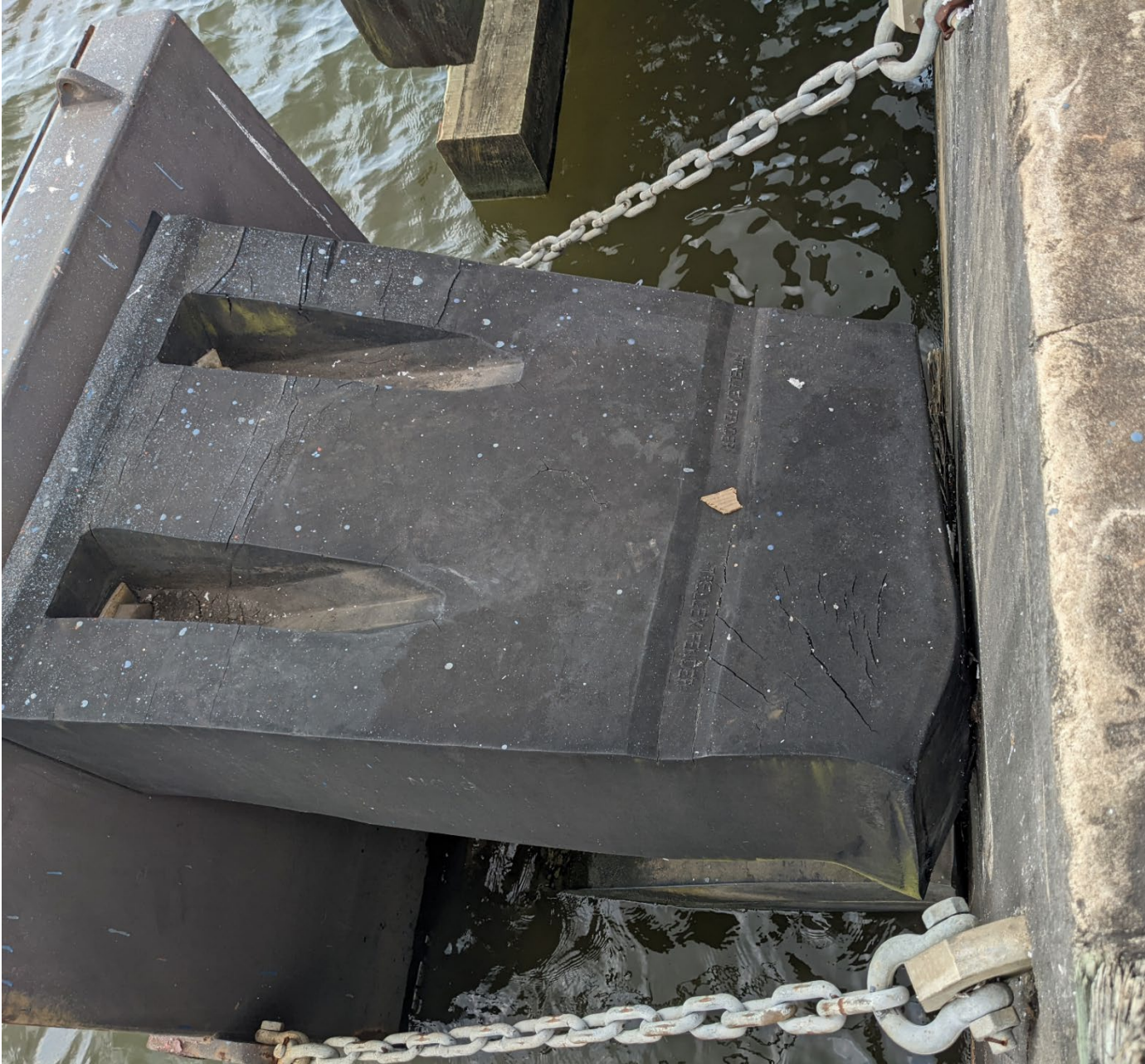
Fender at Cap Log 1087: Replace upper and lower elastomeric rubber elements, including all mounting hardware.
