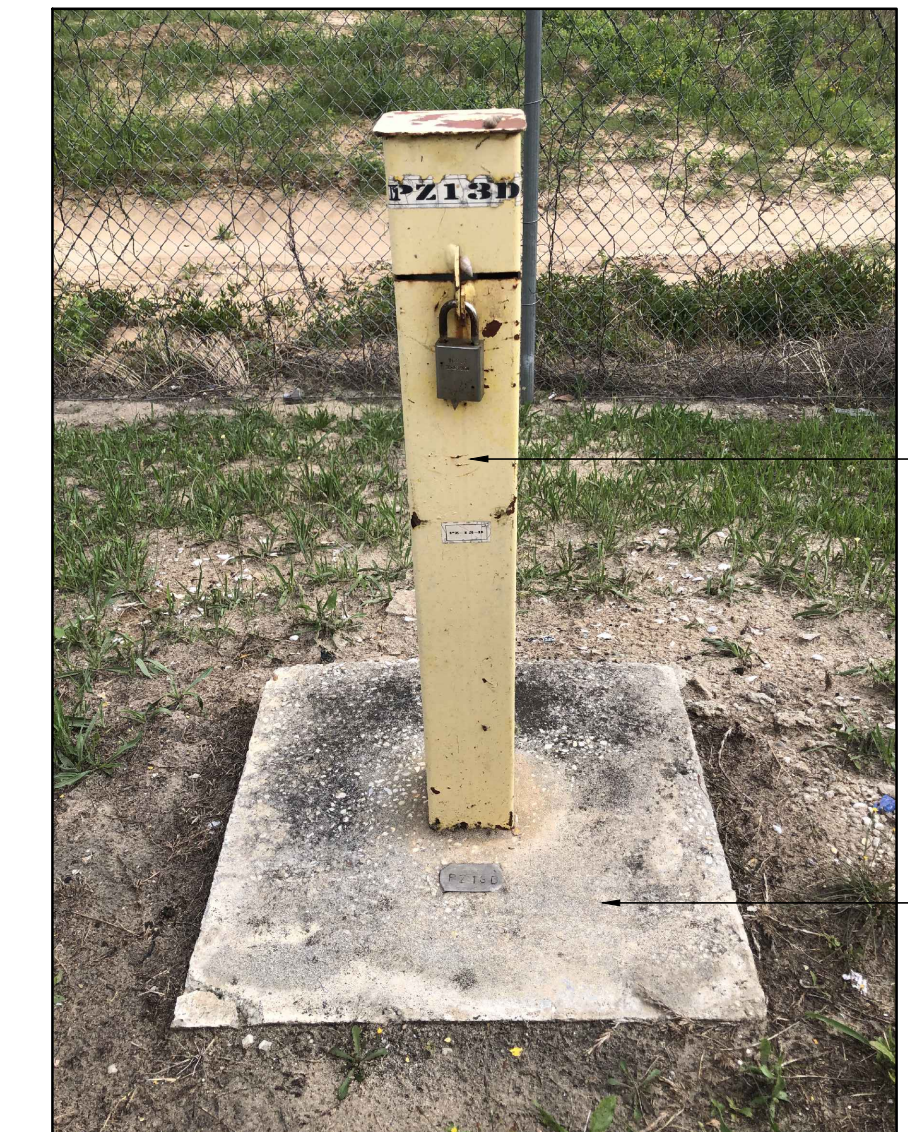
ITEM 1: PIEZOMETER PZ-13-D EXISTING CONDITIONS NTS (VIEW LOOKING NORTH)
