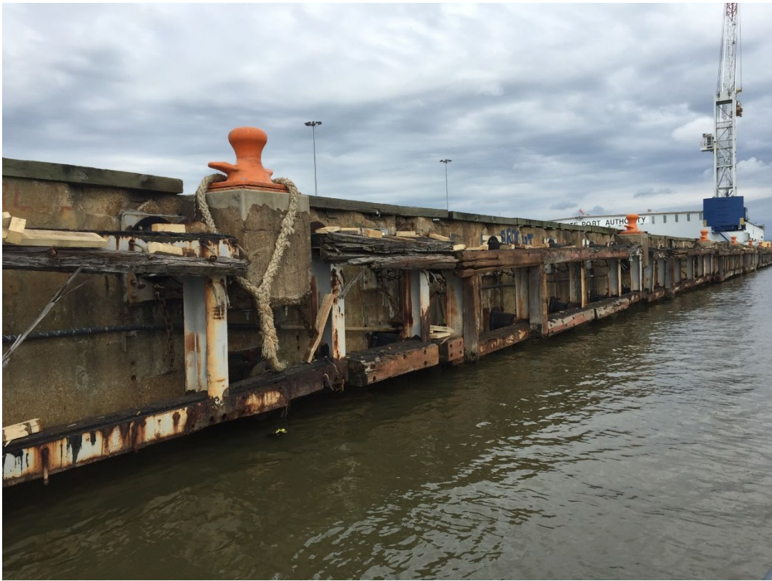
Typical Berth 2 Fender System – Looking Northwest
