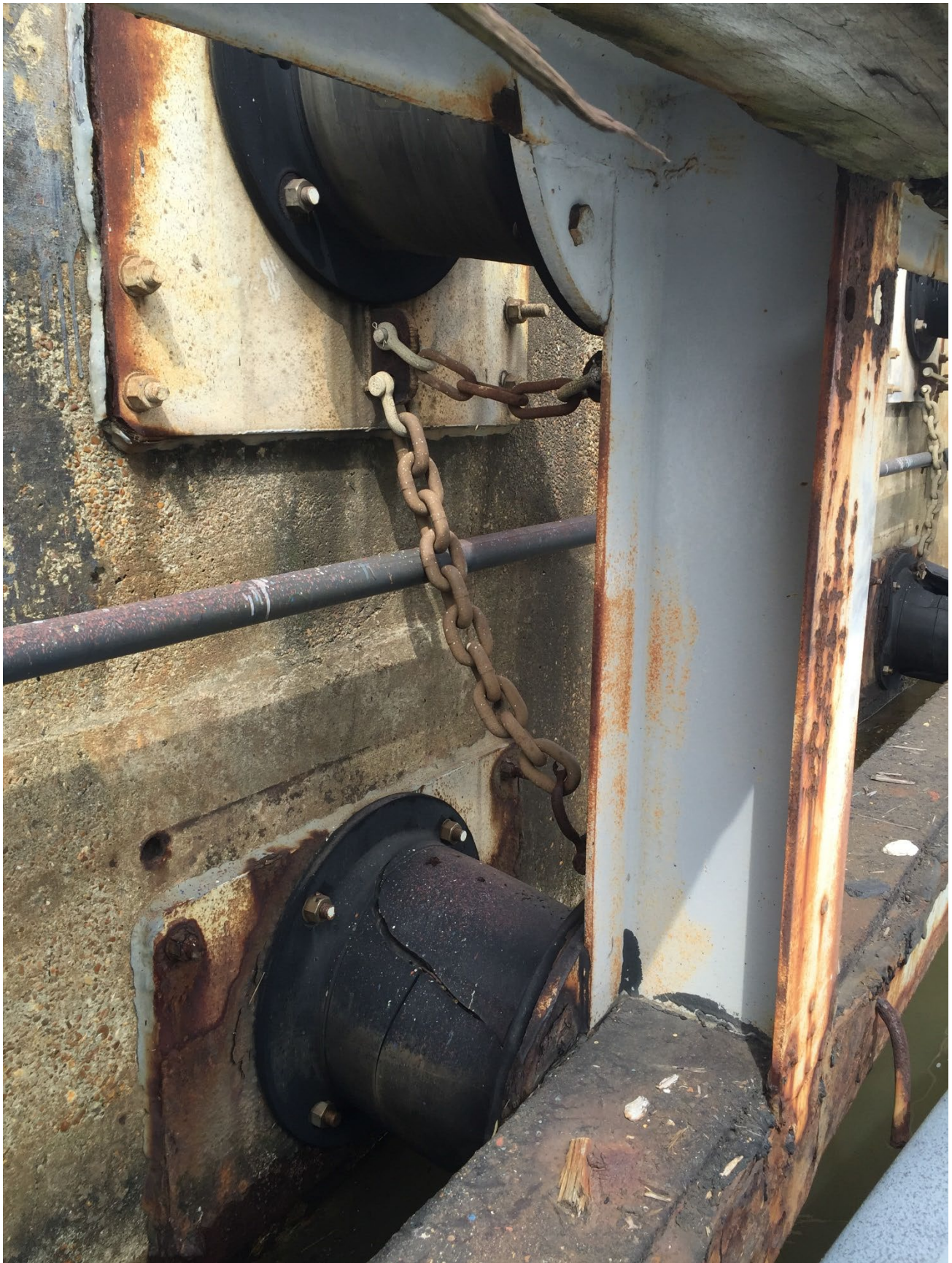
Typical Berth 2 Fender System
