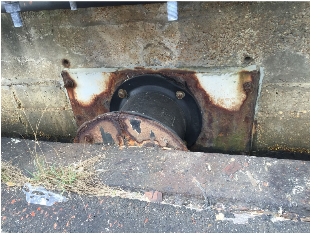
Typical Berth 2 Fender System – Looking West
