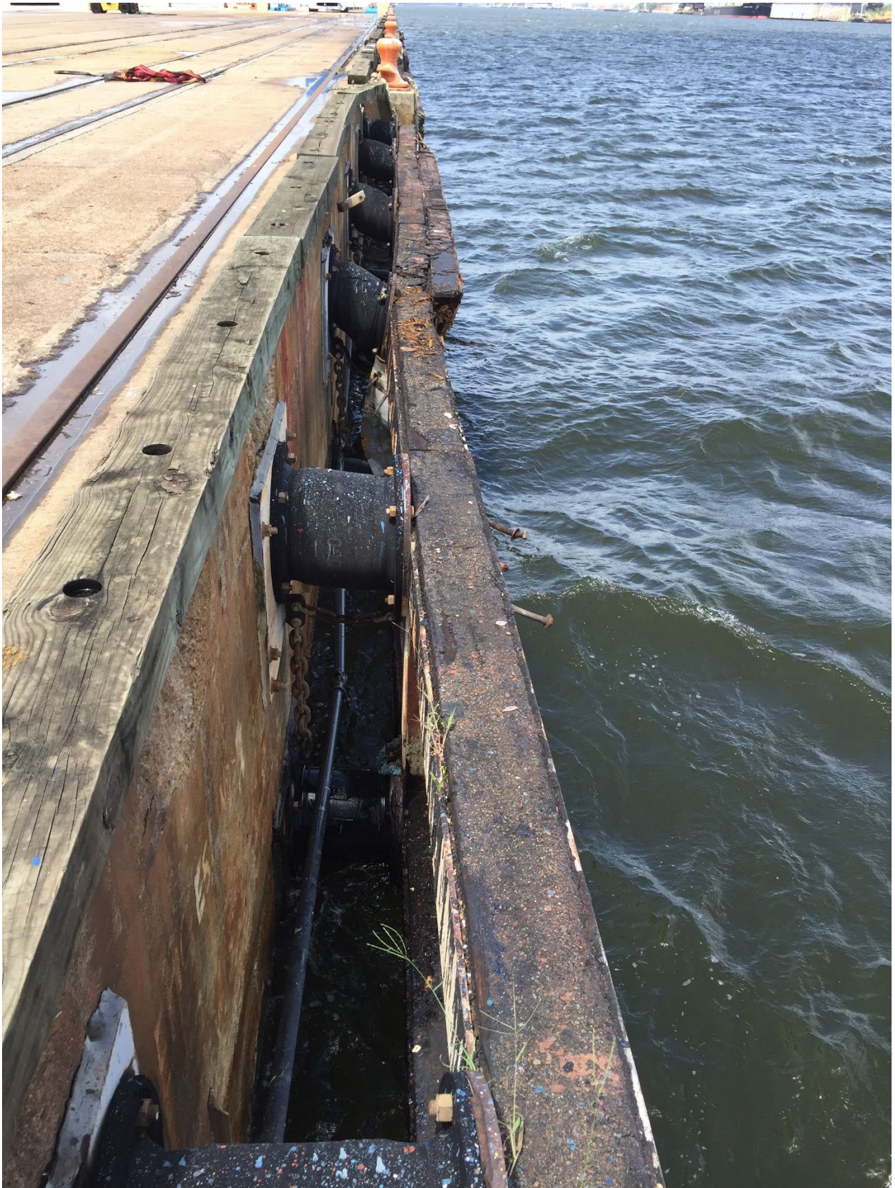
Typical Berth 2 Fender System – Looking North
