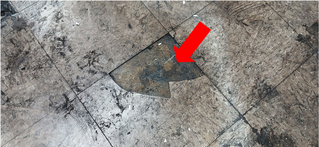
Visual of Inside Building 2 (Warehouse). Office was also found to contain black mastic containing 3% Chrysotile Asbestos underneath VFT.
