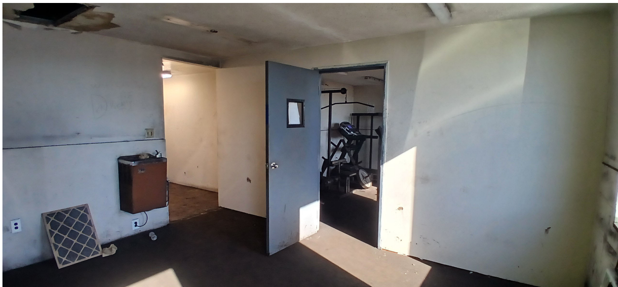
Visual of Inside Building 2 (Warehouse). Weight Room, Kitchen, and Hallway was found to contain black mastic containing 3% Chrysotile Asbestos underneath VFT.
