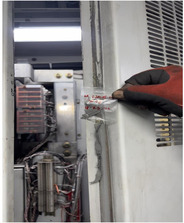
Photo 38 Comments: Suspect Asbestos Sample Collection - Panel Room in Larger Mechanical Room, M Crane
