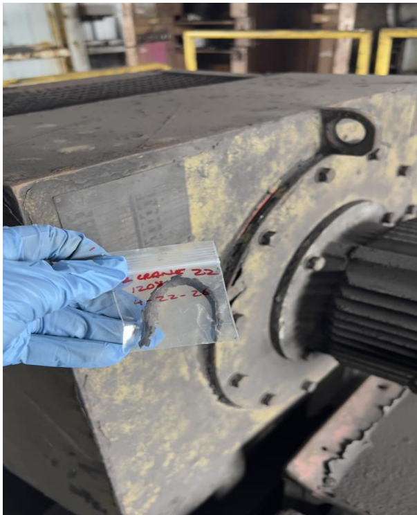
Photo 23 Comments: Suspect Asbestos Sampling - Z Crane Mechanical Room
