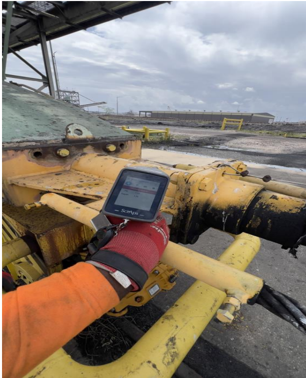
Photo 25 Comments: Lead Paint Inspection Using XRF - M Crane
