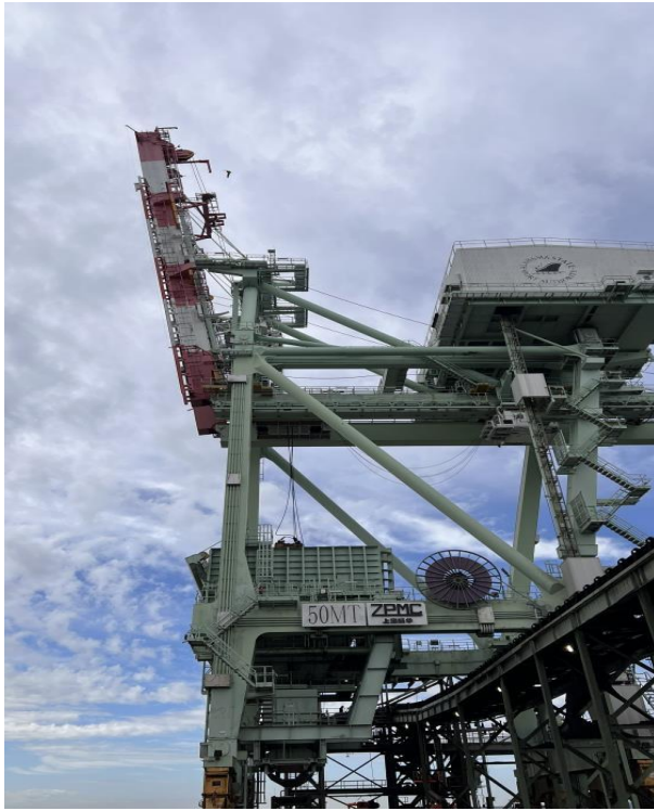
Photo 1 Comments: View of S Crane
