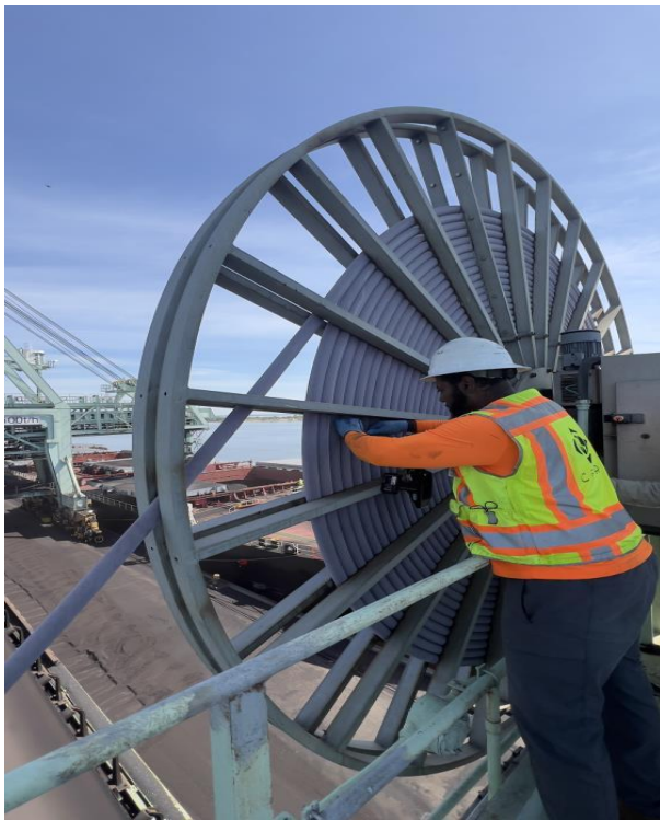
Photo 9 Comments: Suspect Asbestos Sample Collection - S Crane
