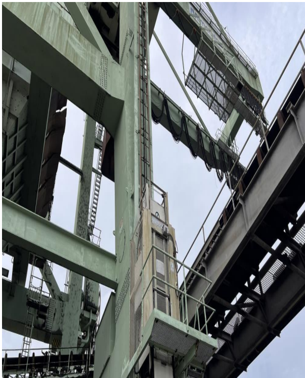
Photo 27 Comments: View of M Crane Elevator
