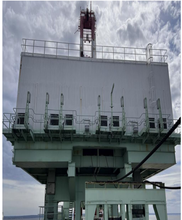
Photo 4 Comments: View of the S Crane Mechanical Room
