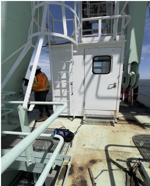
Photo 7 Comments: Boom Control Cabin - S Crane
