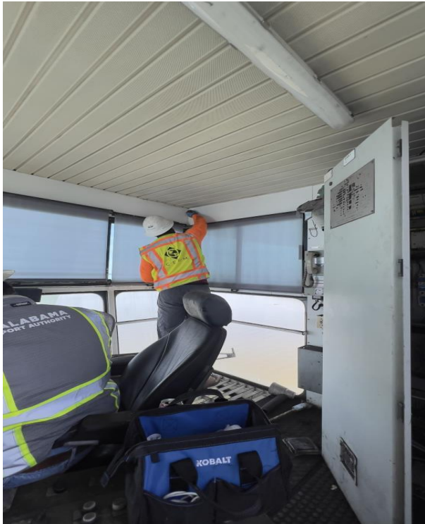
Photo 3 Comments: Suspect Asbestos Sample Collection - S Crane Control Cabin
