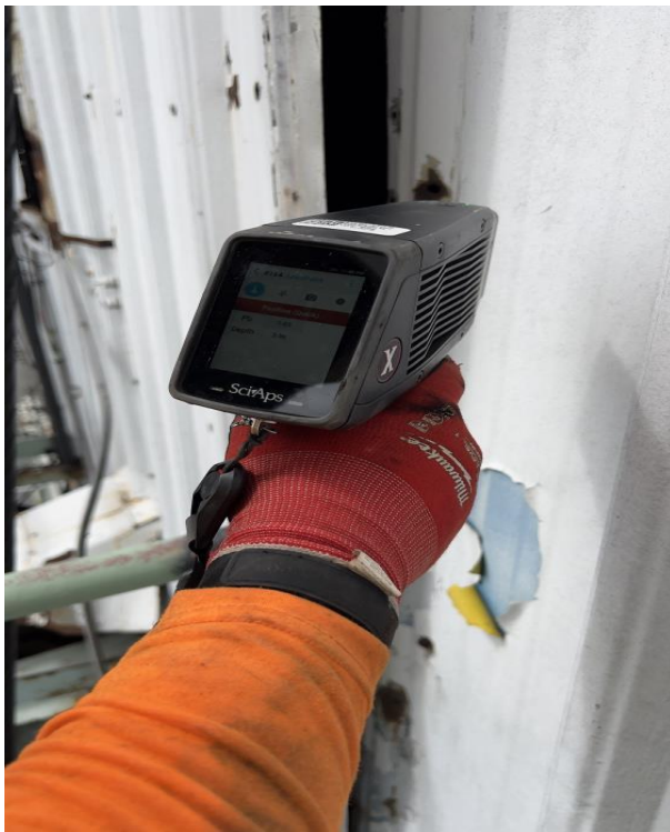
Photo 21 Comments: Lead Paint Inspection - Z Crane Mechanical Room (outer)
