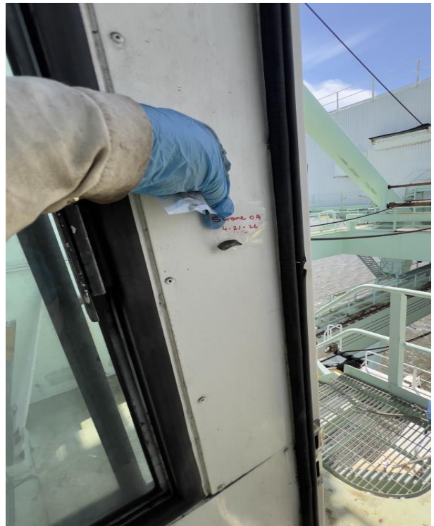
Photo 8 Comments: Suspect Asbestos Sample collection - S Crane Boom Control Cabin
