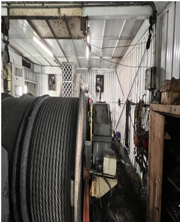
Photo 31 Comments: View of Smaller Mechanical Room (inner)
