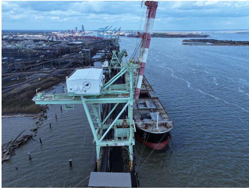
Figure 1: "S" Crane looking north
