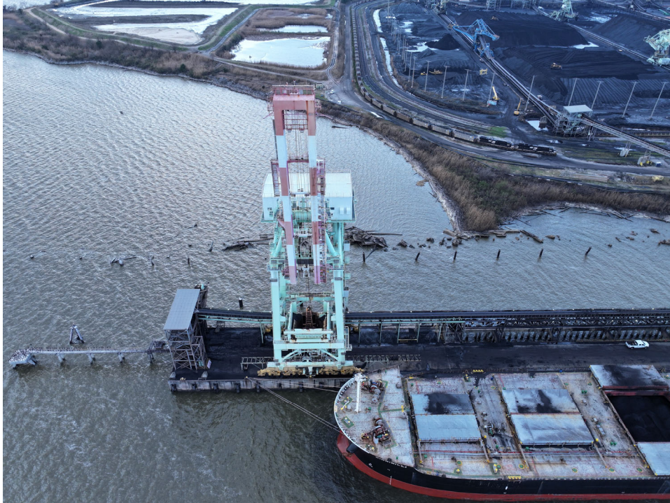
Figure 3: "S" Crane looking west
