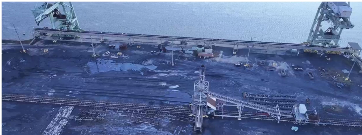
Figure 9: Yard 4 west of "M" and "Z" Cranes
