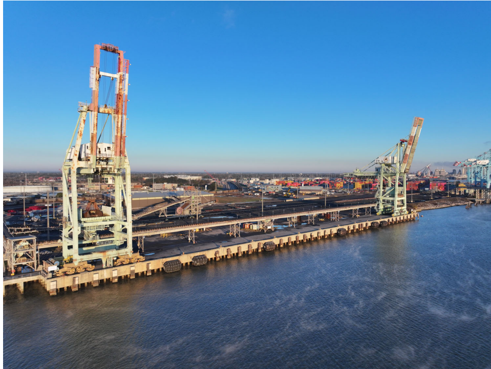
Figure 5: "Z" Crane on the left and "M" Crane on the right
