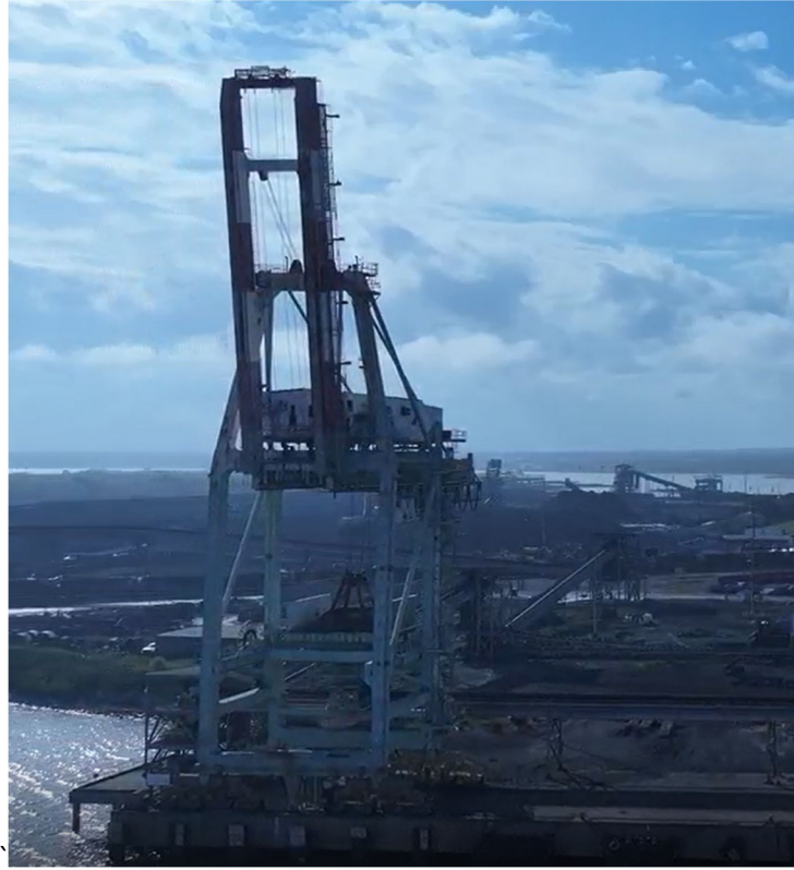
Figure 8: "Z" Crane looking west
