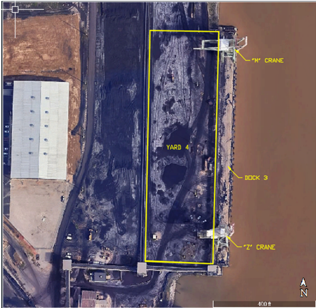
Figure 12: Yard 4 Work Area
