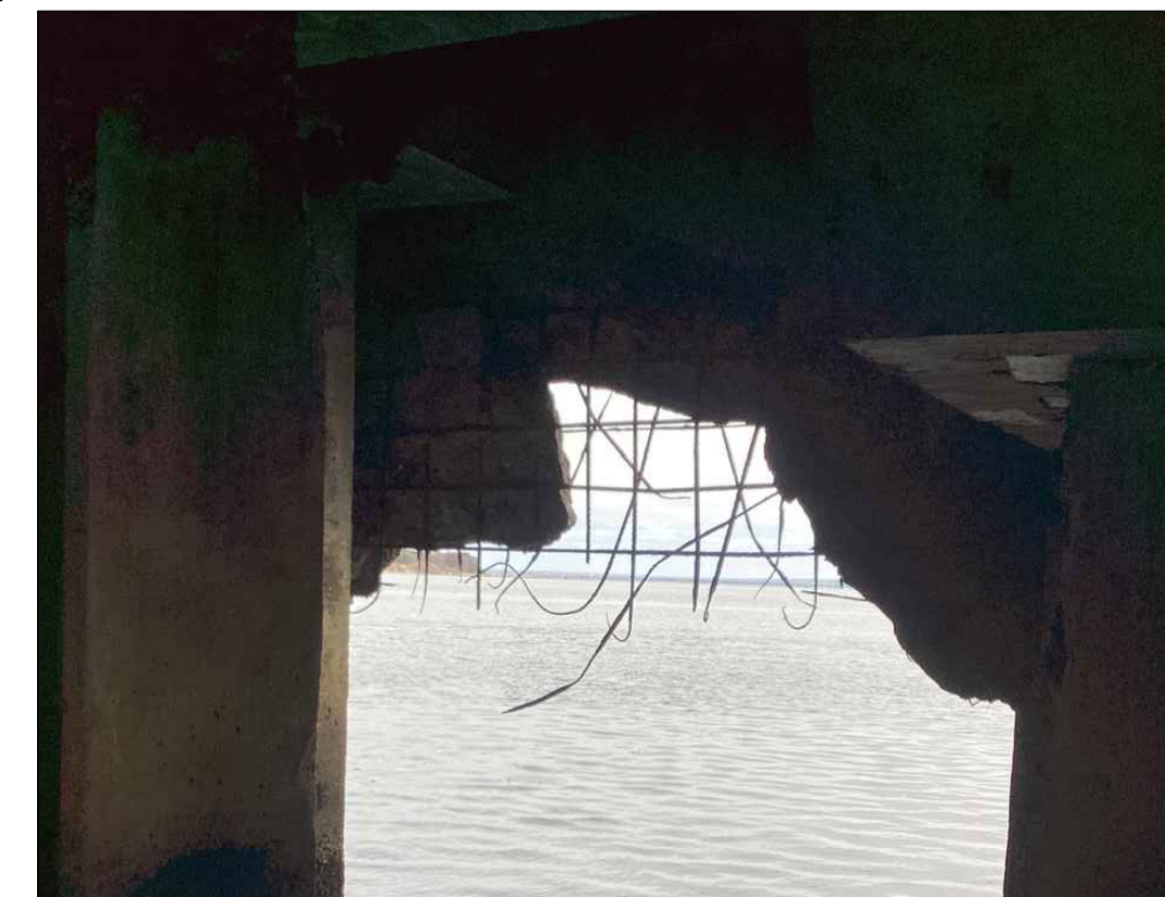
WALL DAMAGE REFERENCE PHOTO @ LOCATION 54 N.T.S.
